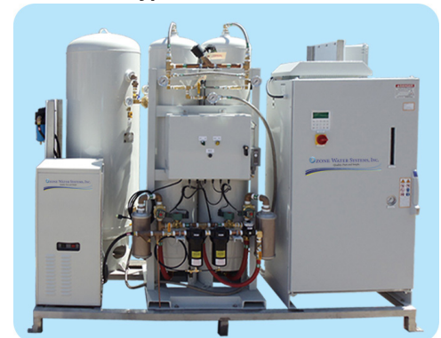
Typical Ozone Skid
